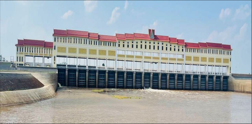
Raksa Hydropower Dam started construction in 2019, upstream of the watershed, can store 256.9 million m3 during the rainy season.
