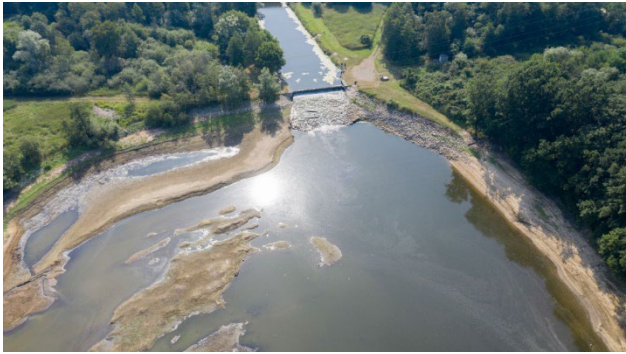
Low water level at Hullern reservoir, 2019 (Gelsenwasser)
