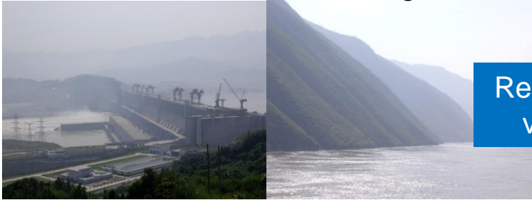
Construction of the Three Gorges Dam
