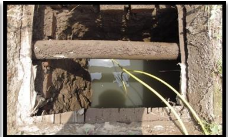
Sumur resapan Perhutani Area
