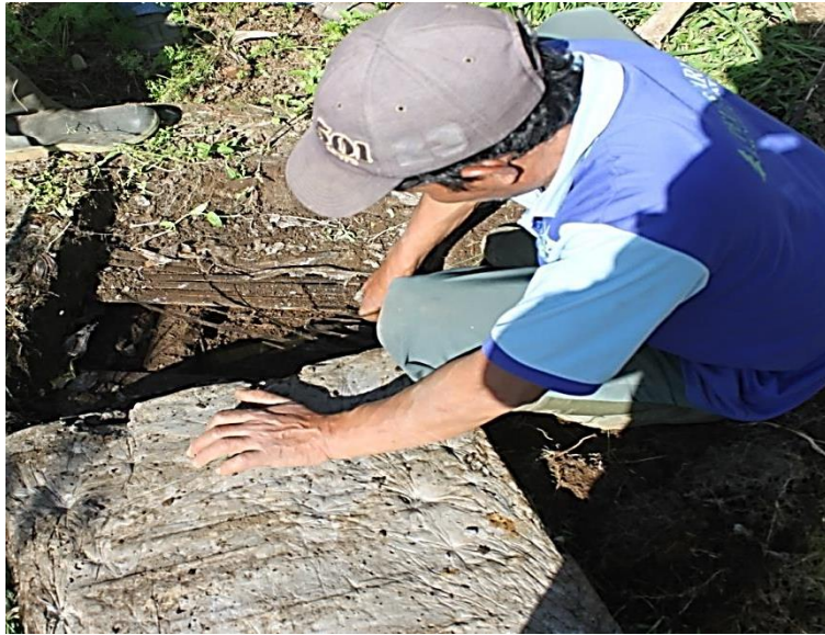
Infiltration pond at agricultural land. Control box was filled by sediment (Padusan Village, Mojokerto)
