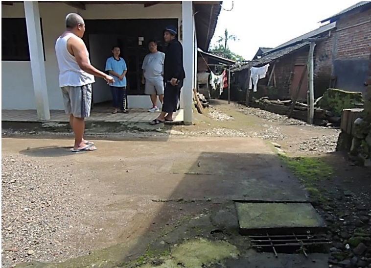
Infiltration pond at residential area in good condition (Claket Village, Mojokerto)
