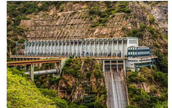
Fig 3. Hydroelectric Power Plant Mantaro(From Google Photos)
